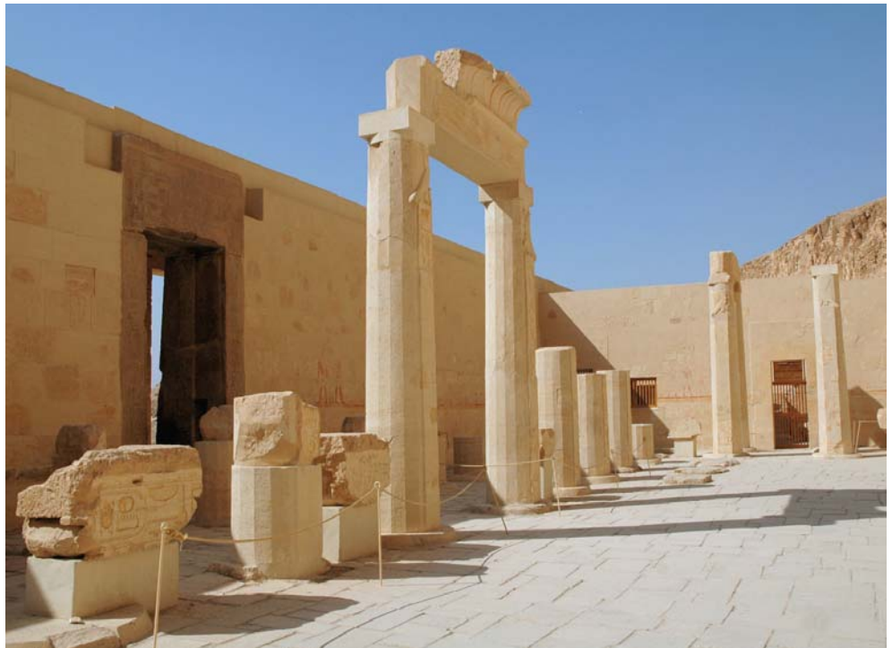
Fig. 1. Upper Courtyard looking towards southeast corner. Polygonal columns have been restored to various heights depending on the number of ancient fragments they contain. Some fragments of architraves are set on plinths (left front).
