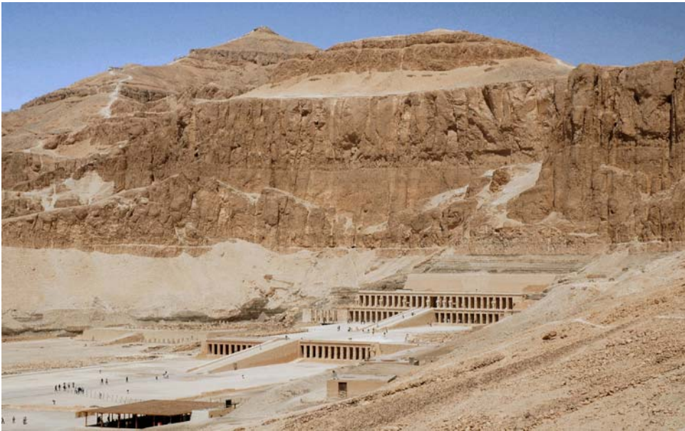
Fig. 2. Hatshepsut's Mortuary Temple at Deir el-Bahri lies beneath unstable cliffs of shale topped by massive limestone.
